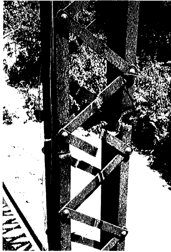
Fig. 41. Photograph of damaged member after collapsing upon itself.
