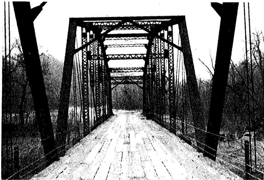
Fig. 1. Photographs of the Hubby Bridge.
