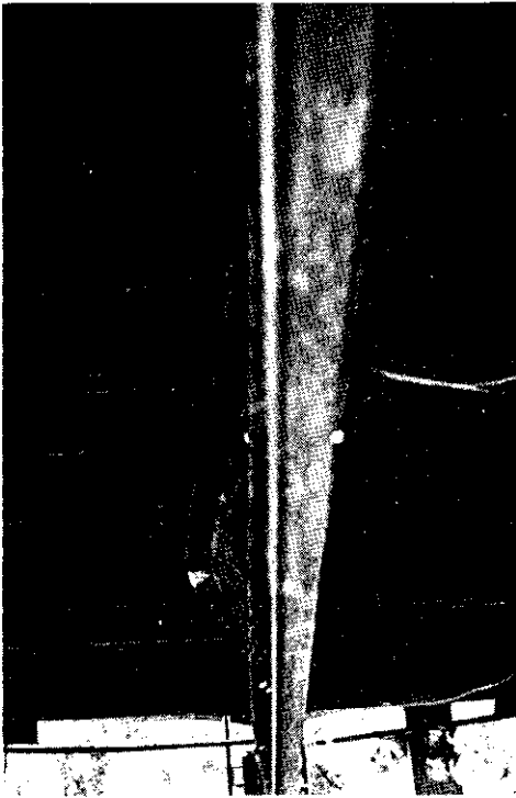
Fig. 48. Photograph of buckling of compression flange of floorbeam 5.
