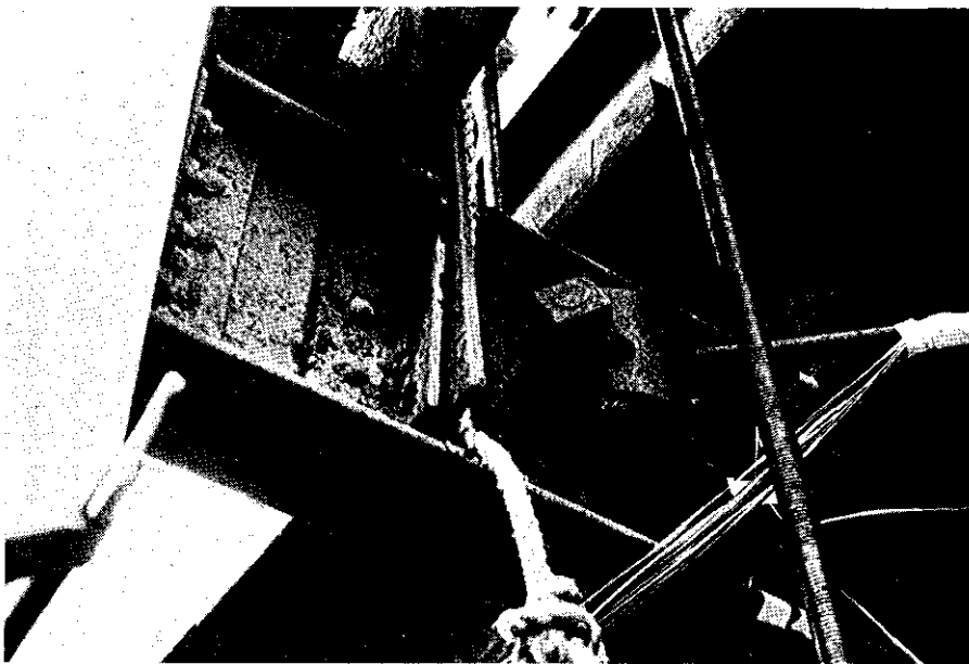
Fig. 52. Photograph showing where last four bolts broke.
