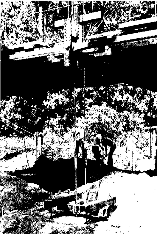
Fig. 26. Photograph showing system used to attach steel rods to concrete mats.
